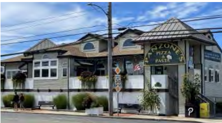
Renovated restaurant, 1106 N Bay Ave. at Ninth St.
