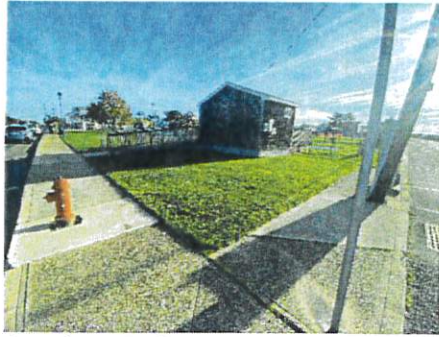
At point 1 facing East.
